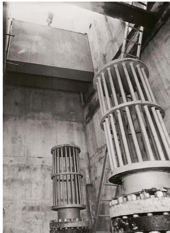
The above photograph shows a silencer under construction designed to vent 620,000 Nm<sup>3</sup>/hr of natural gas to atmosphere from 76 bar.
