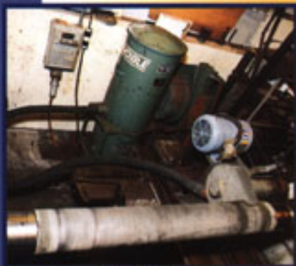
Still going strong. This lathe generates large amounts of chips and airborne dust while machining rubber rolls. An older INVINCIBLE machine purchased in 1984 and formerly used for housekeeping was connected to a custom-fit source capture collection hood. Results — a cleaner, healthier work environment and improved working conditions.
