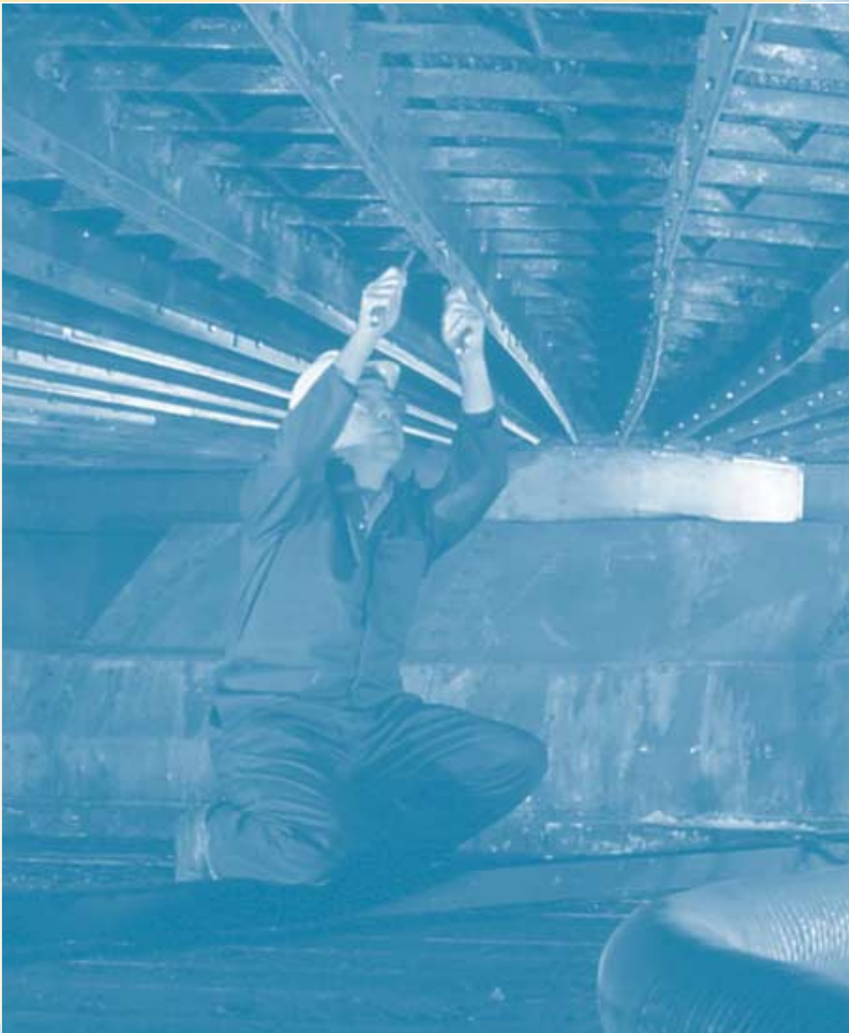
Air preheater sealing enhancement nearing completion
