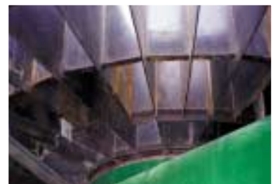
Retrofitting the Howden sealing system can substantially reduce air preheater leakage
