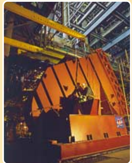
In some instances the installation of a new fan can be economically justified
