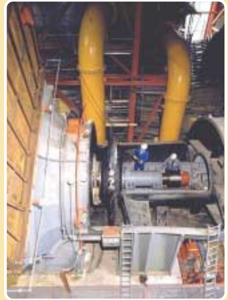
Replacing blades or the complete rotating assembly can significantly increase output or reduce power consumption
